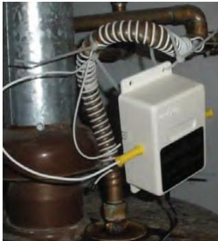
An Aqua-Rex WK1 was installed on the flexible cold water connection to the tank water heater and plugged into a nearby outlet. The signal generated by the Aqua-Rex travels through the water into the heater & also travels back against the flow to treat all the cold water in the property.
